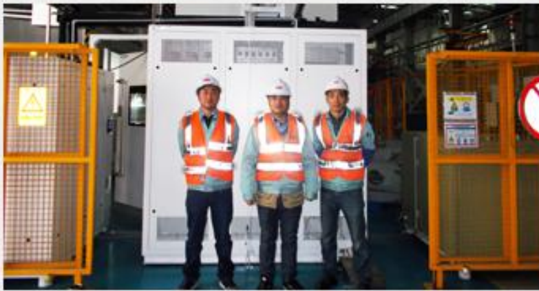
► On-site Installation for ABB
