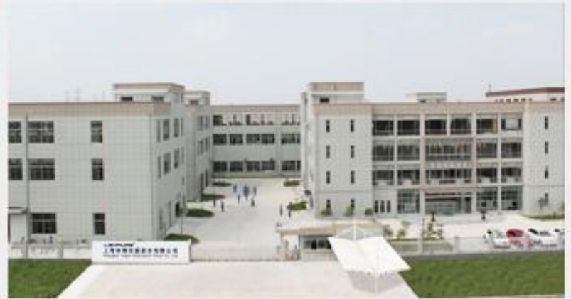
► With 5 buildings for Various Departments
